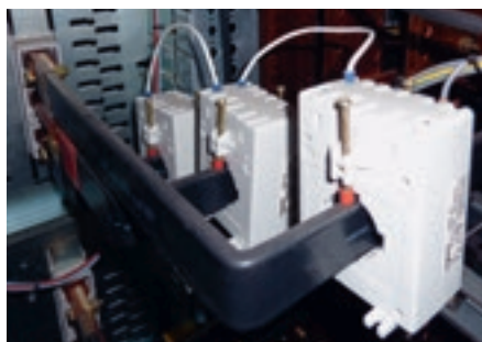
Current transformers mounted directly on flexible busbars
