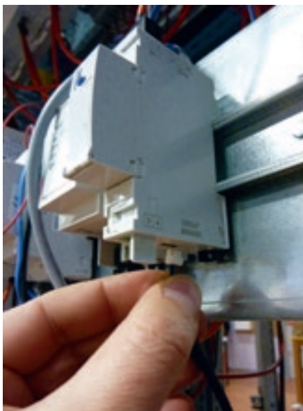
Connection under the communication interface. The connecting cable is supplied with the interface.
